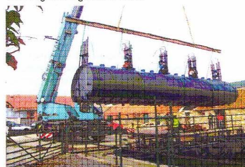
Set of Organic Power tanks being loaded into a lagoon
